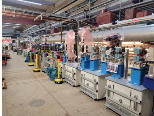
Installation of new LH section
