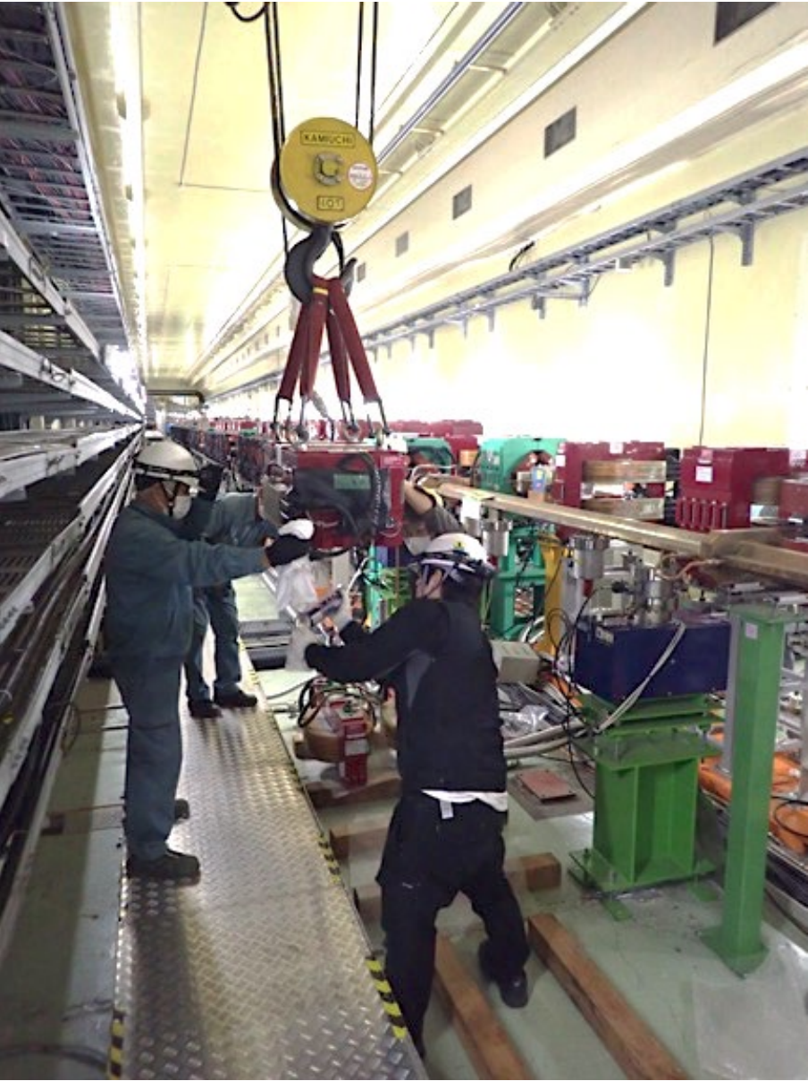
Dividing wigger magnets to remove a beam pipe
