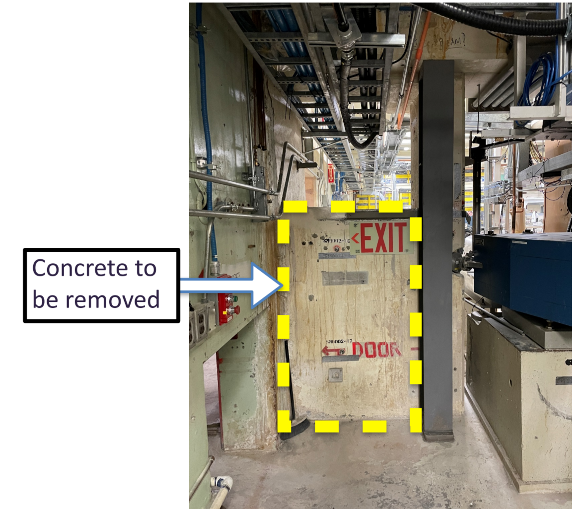
Figure 9. Shielding wall at end of linac.
