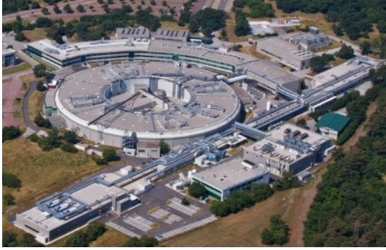
Elettra (2 and 2.4 GeV) - Italy
